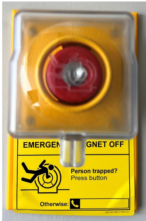
Figure 4. The WSU CoNNECT is fitted with two Emergency RUNDOWN switches. One is located near the control station (Zone III) and the other is in the MRI room (Zone IV).
