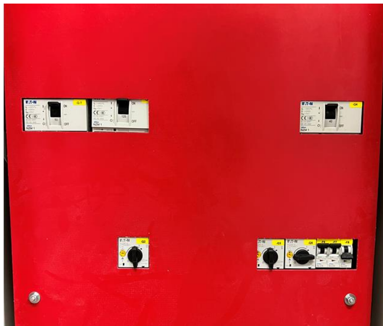
Figure 3. Philips dStream Achieva 3.0T gMDU located in the MRI Equipment Room (Zone III).
